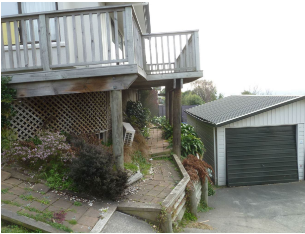
Figure 1: Tilting pole structure
