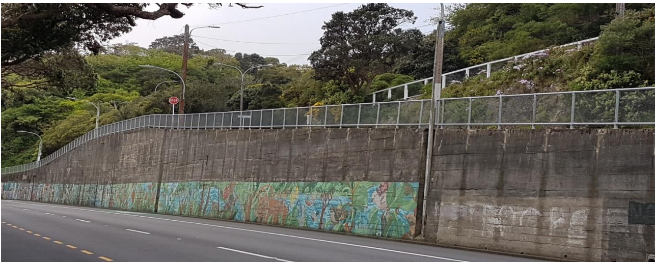
Figure 2.1: Retaining Walls along Chaytor Street
