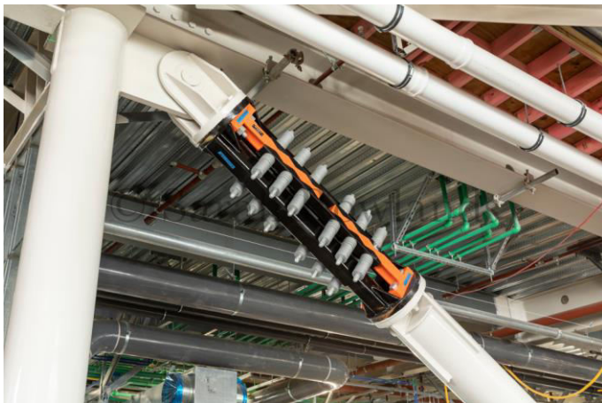
Figure 12 –RSFJ Brace Assembly (RBA)
