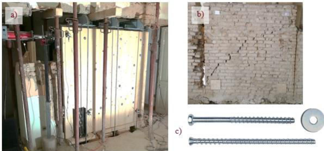
Figure 7: Full-scale tests: a) Reinforced wall with CLT panel ready to be tested [11], b) Stair-stepped failure observed after testing, c) Dry fasteners used for the CLT panel-to-masonry wall connection
