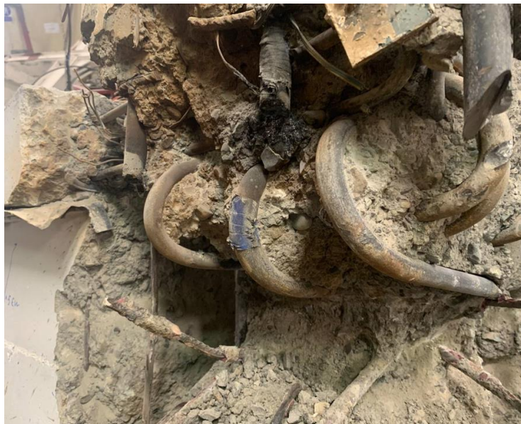
Figure 8: The beam-column joint after demolition
