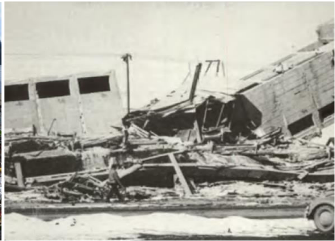
Figure 2: The collapsed Four Seasons Apartments after the 1964 Anchorage (USA) earthquake
