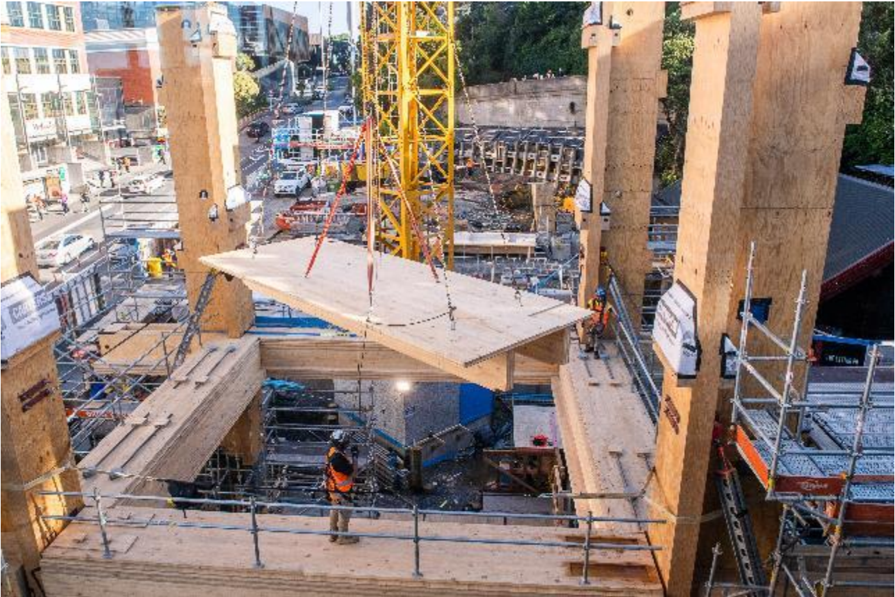
Figure 8: Installation of prefabricated 'double T' floor panel
