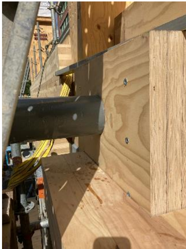
Figure 7: 150 diameter steel pin installation
