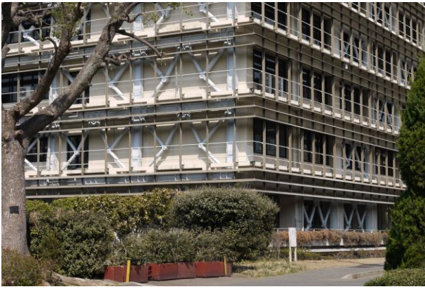
Figure 11: Governmental Building in Japan with Toggle-Brace-Dampers
