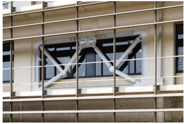
Figure 11: Governmental Building in Japan with Toggle-Brace-Dampers
